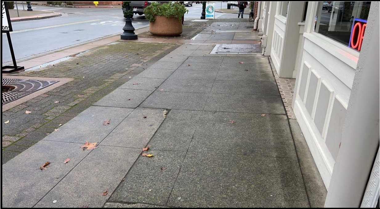
Figure 1: Existing Sidewalk on Montgomery Street
